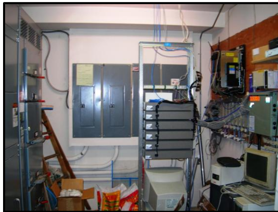
Remove all storage items from electrical room
