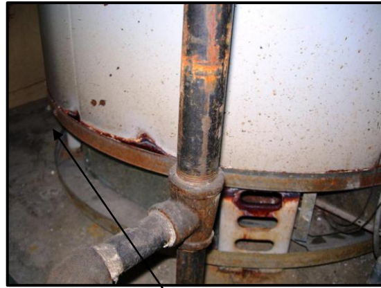
Water heater #3 is leaking
