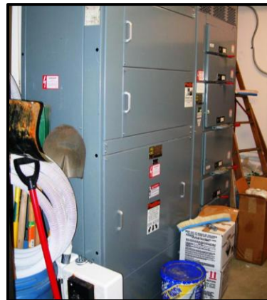
Remove all storage items from electrical room
