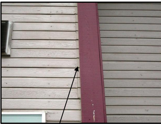
Siding was cut too short (poor installation)
