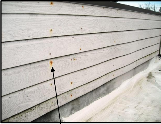
Siding on the parapet walls needs to be replaced
