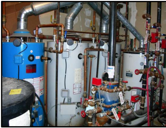
General view of the water heaters
