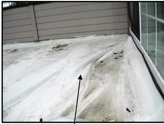
Rippled roofing material (poorly installed)
