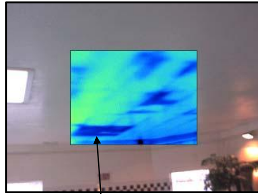
Thermal Scan of pool ceiling (blue areas were verified as wet)
