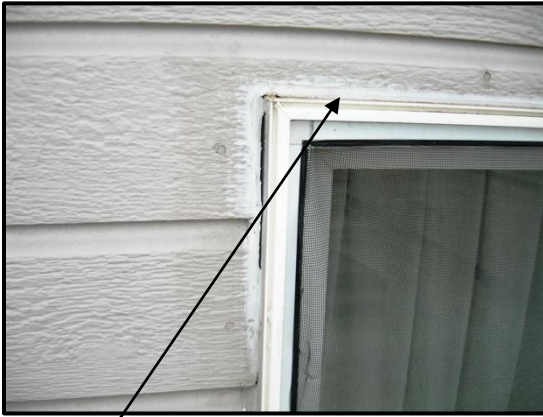
No flashing above the windows
